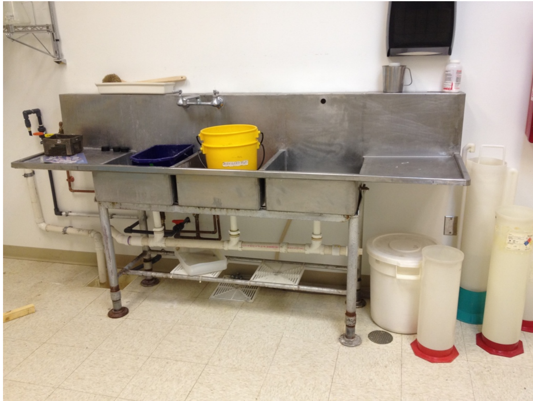
Three bowl sink with right and left drain boards Bowl Size: 17" W x 17" L x 7"D Overall: 92" W x 24" L
